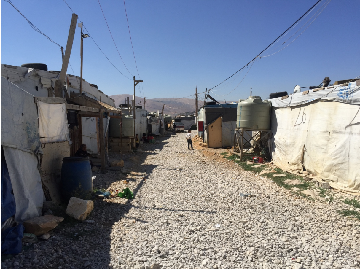
Figure 2. Quality of shelter units in one of the Syrian refugee encampments in Bekaa. Photo by Marwa Abou Zeinab, LESS
